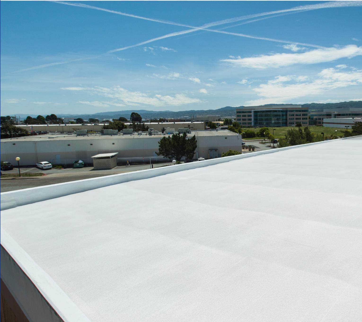
**KM Coatings'** spray-applied polyurethane foam (SPF) roof systems offer sustainability and high performance. No seams, no fasteners, self-flashing system that can be re-coated and renewed to extend the life of the roof. The highly reflective top coat surface works with the insulation to reduce roof temperatures and thermal stress. This system eliminates thermal bridging, adds superior insulation properties for improved building energy efficiency and indoor environment.
